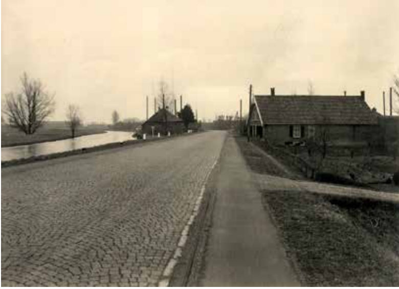
Figure 10 Traffic separation was not possible everywhere in the Dutch landscape but getting cyclists off the main road remained a priority. This provincial sand road between De Meern and Oudewater in Utrecht province was paved somewhere between 1924 and 1934. The adjacent asphalt lanes were intended to “seduce” cyclists into not riding in the middle of the road. [Source: Collectie Het Utrechts Archief, Photographer: Jochmann Disco, no. 220755]
