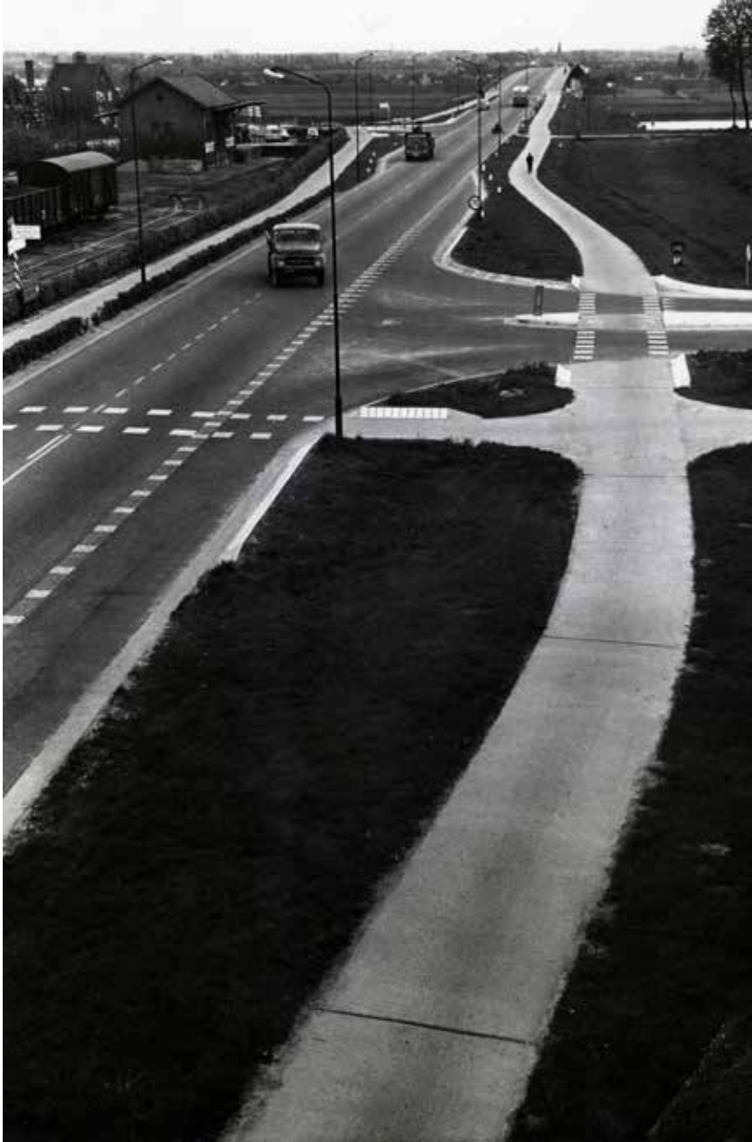
Figure 20 Provincial engineers constructed cycling paths in part to accommodate moped riders. They believed widening and expanding the cycle path network was crucial given the considerable cohort of Dutch commuter cyclists. This path was built between 1955 and 1960 near Rhenen, Utrecht province, at a time when only a few countries were still constructing (utilitarian) cycling infrastructure [Source: Photographer Provincie Utrecht, Collectie Het Utrechts Archief, no. 837959]
