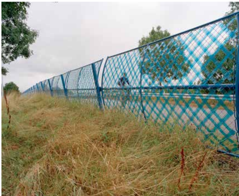
Figure 32 This (ultimately unsuccessful) experiment with a wind protection screen along a bridge was part of the Bicycle Masterplan, a policy document devised in the 1990s. It illustrates how with this plan and since then, the Dutch national government has encouraged and boosted innovation and knowledge production in cycling, leaving the implementation of pro-cycling and car-limiting measures mostly to local government. [Source: Collectie Het Utrechts Archief, Fotodienst GAU, no. 823903]
