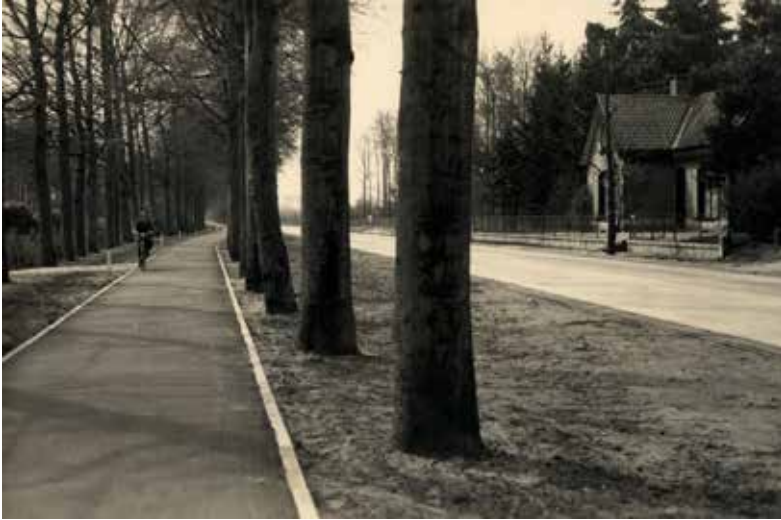
Figure 8 National engineers' ideal was to separate cyclists and car drivers completely. At this provincial road between Soestdijk and Bilthoven, Utrecht province, the engineers achieved that (c. 1930) by turning the former road into a cycling path while constructing a new road to the right of the row of trees. [Source: Collectie Het Utrechts Archief, Photographer unknown, no. 220773]
