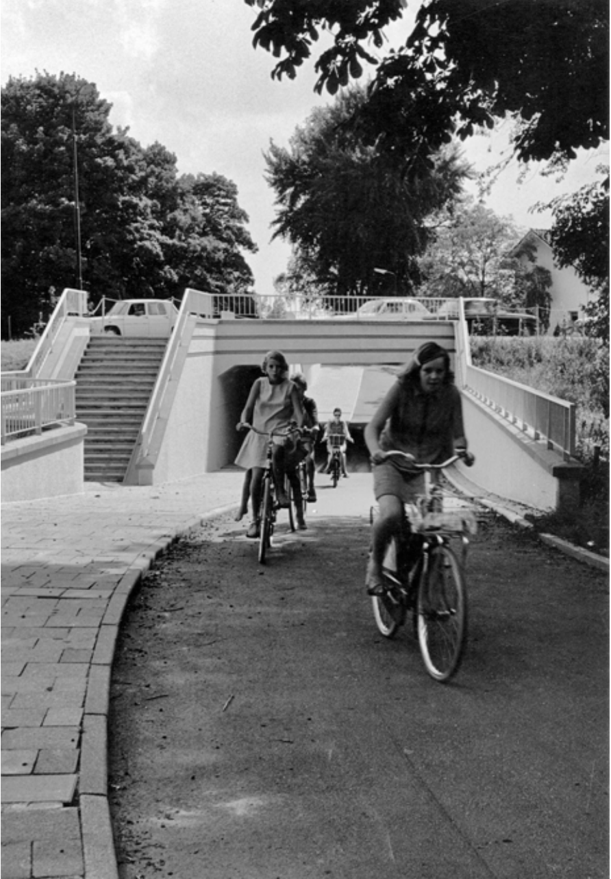
Figure 31 Cycling tunnels like these near Vreeland, Utrecht, enabled cyclists to cross larger roads safely and prevent detours, making cycling a more attractive option. Since the 1970s, cities increasingly invested in such tunnels in response to broad public demand for cycling and safety. Part of the budget came from national governmental subsidies. [Source: Collectie HUA, fotograaf Provincie Utrecht, nr. 847441]
