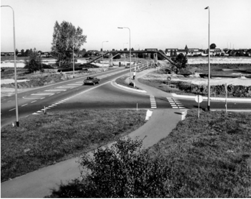
Figure 17 The Dutch ANWB increasingly promoted driving over the 1950s and 1960s, and sought to maintain cycling, believing it could simultaneously facilitate both. This junction near De Meern, Utrecht in 1975, developed by ANWB experts in the 1950s, has been widely applied since then to prevent collisions between cars turning and cyclists crossing. The ANWB circulated its design ideas among engineers through its trade journals, engineering courses, and good contacts with authorities. [Source: Collectie Het Utrechts Archief, Photograph Provincie Utrecht 847432]
